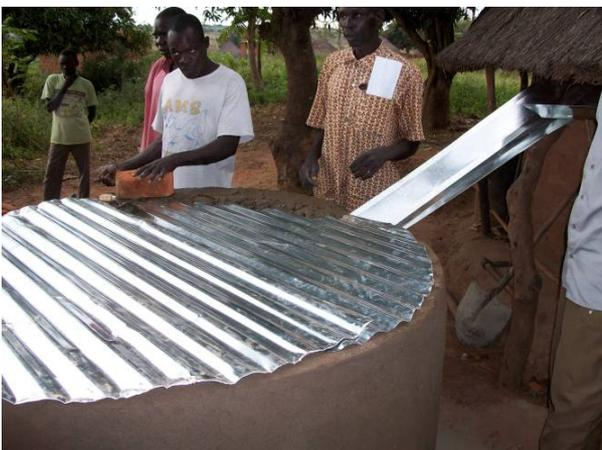
The lid of the tank has to provide a long-lasting cover against sunlight, insects and debris entering the collected water, whilst being removable to allow removal of the water. This is particularly important in areas where malaria is present, as the tanks would otherwise become mosquito breeding centres.
