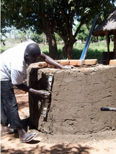
The DRIP tank is a fired brick built cylindrical tank standing on a base of approximately 1.5m diameter.
