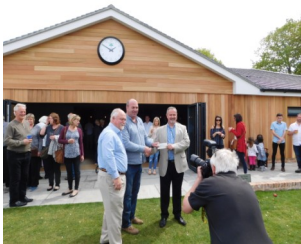
Accessible toilet in the new Rainham Cricket Club pavilion
